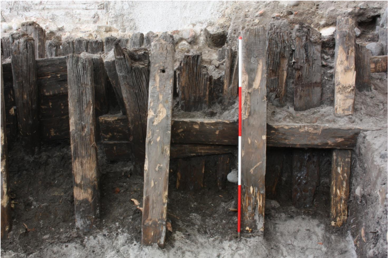
Fig. 64 Close up of harbour bulwark G648 next to the baulk. The photo is centered on an area of repair shown by horizontal plank ST41884 and three vertically set planks (ST39435, ST39413, ST55582) used as the plank's support. The photo is looking N. C03_20140613_10920
