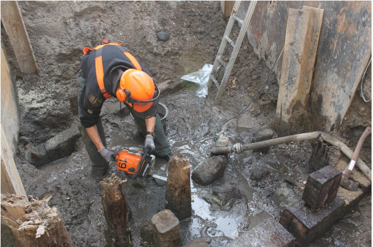
Fig. 182 Photo displaying the use of chainsaw cutting the timbers for analysis. Guide Wall excavation 2012. C19_20121018_4271
